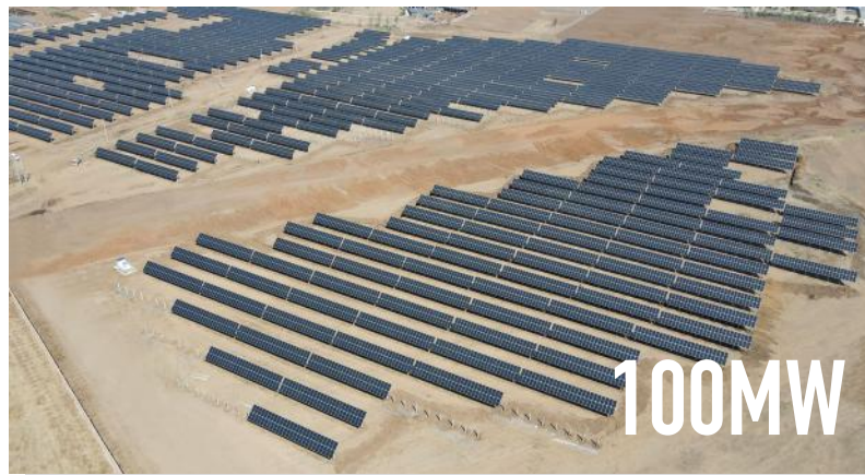
Project Type: G-Mounted Location: China / Liaoning Commission Date: 2021-11 Product: SRP-405-BMD-HV
