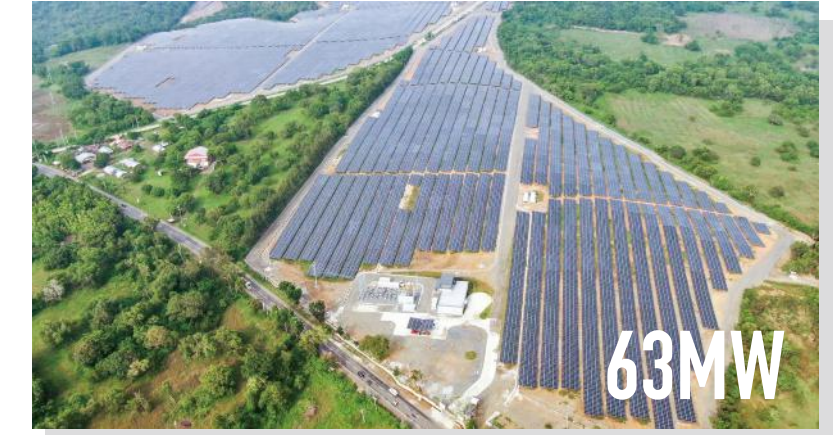
Project Type: G-Mounted Location: Philippines / Zambales Commission Date: 2021-3 Product: SRP-400 / 405-BMD-HV
