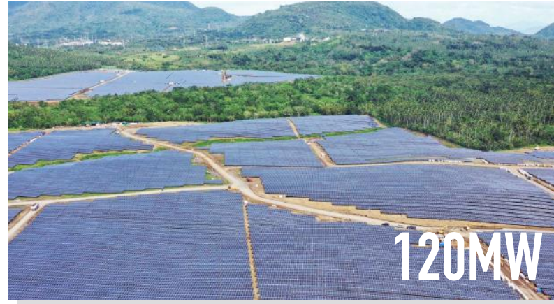
Project Type: G-Mounted Location: Philippines / Laguna Commission Date: 2021-6 Product: SRP-405-BMD-HV
